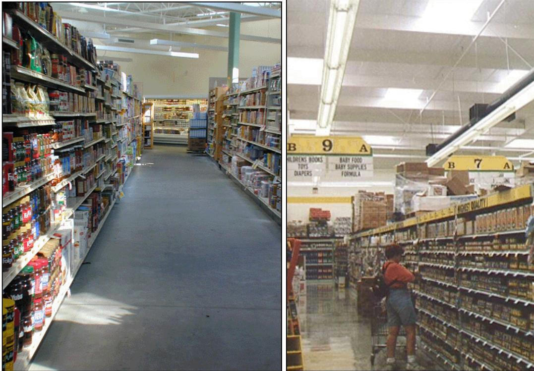
Figure 9. Clear skylight with “hot spot” and diffuse skylights with even lighting
